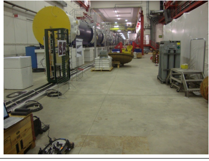
(b) ECN3 tunnel at CERN
